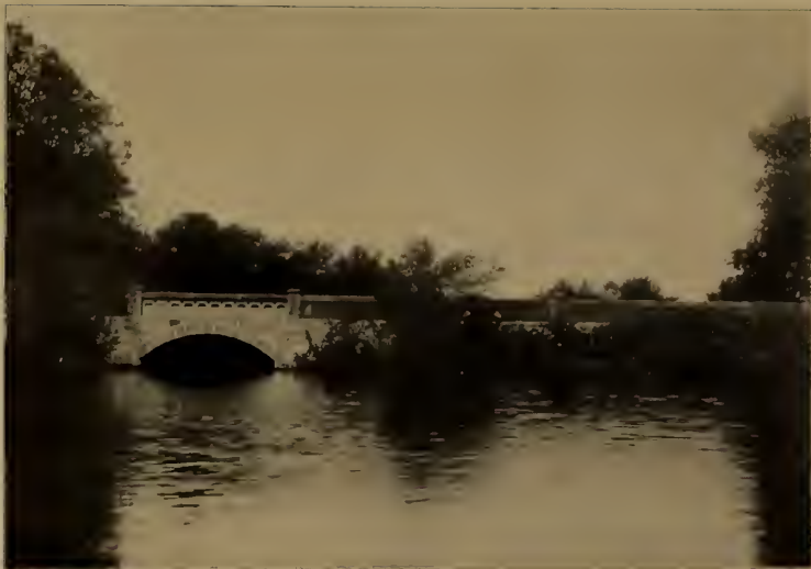
BRIDGE AT LANGWATER, ESTATE OF MRS. FREDERICK L. AMES, North Easton, Mass.
